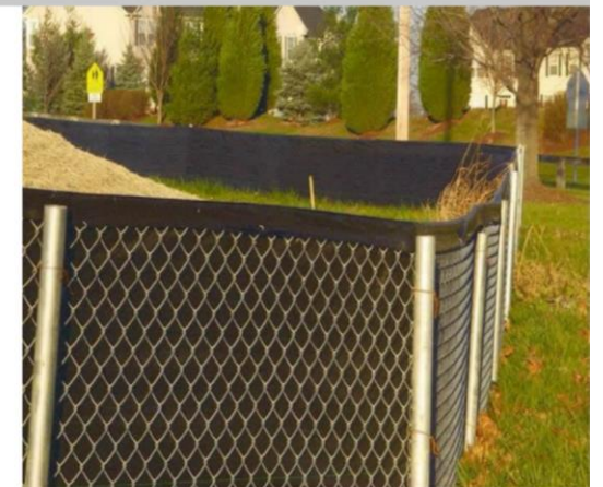
Super Silt Fence Details and Installation Photo
