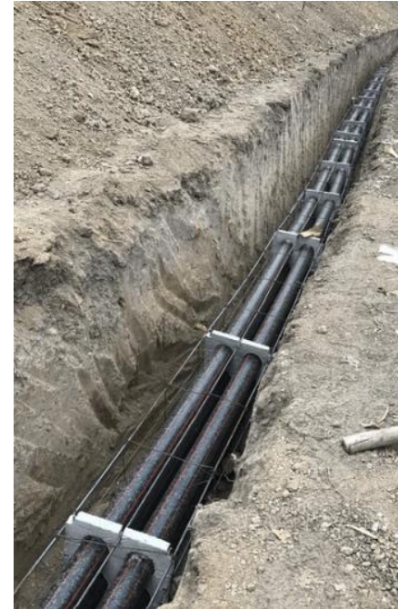
Example of underground conduit lines.
