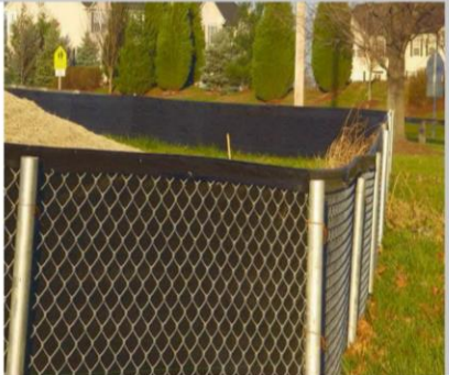
Super Silt Fence Details
