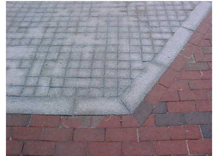
GRANITE HC RAMP PAVERS
